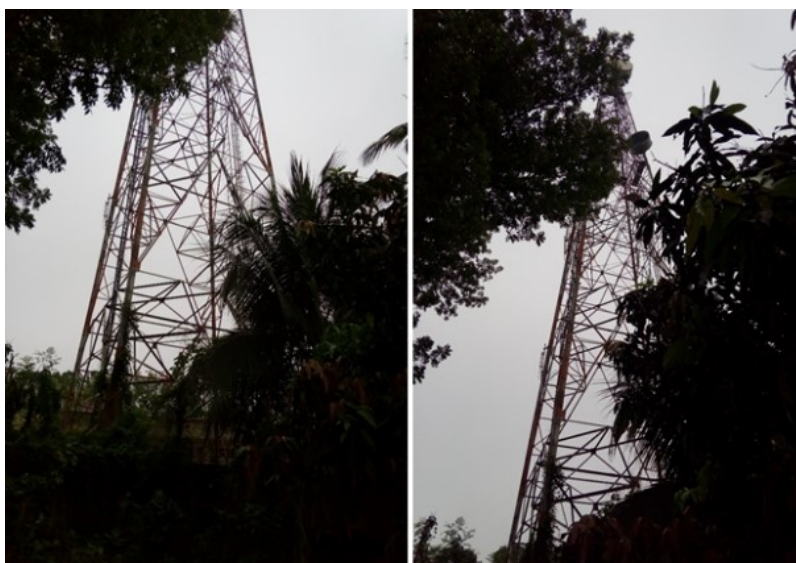
Figure 1 Cellular Base Transceiver Station (BTS) in Burdwan, West Bengal
